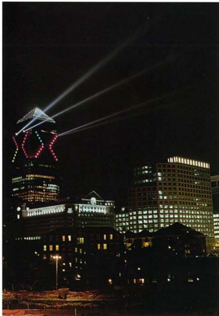
Aimed at the City - west-facing xenon STX skylights 'putting their best beams forward.'
